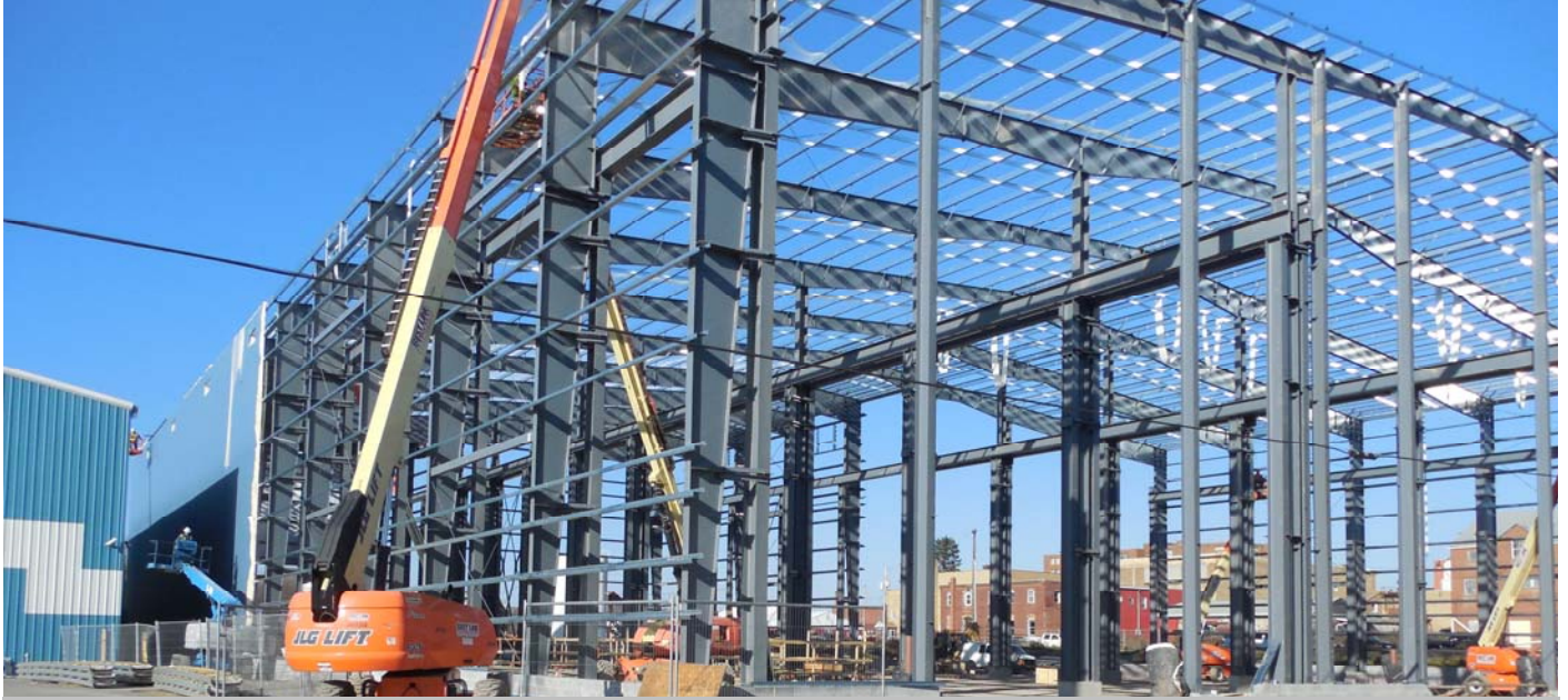
Lee Industries – Expansion Project
