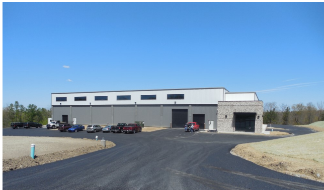
Diamondback Automotive Accessories - Construction nearing completion.
