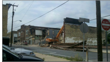
Guenot Building on East Pine Street
